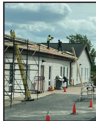
One project worked on was the CIA#3 Roof Replacement.
